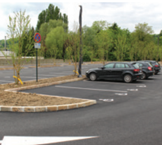
Parking, avenue Paul Thoureau
